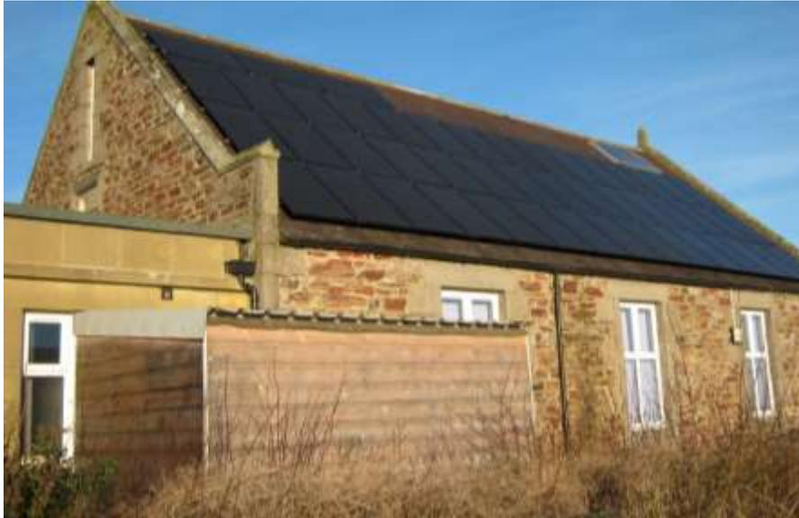
*“The grant contributed to a solar panel array at the Newmill Hall. This complements our biomass boiler as some of the electricity is used to power the electric pumps which the boiler requires.*
