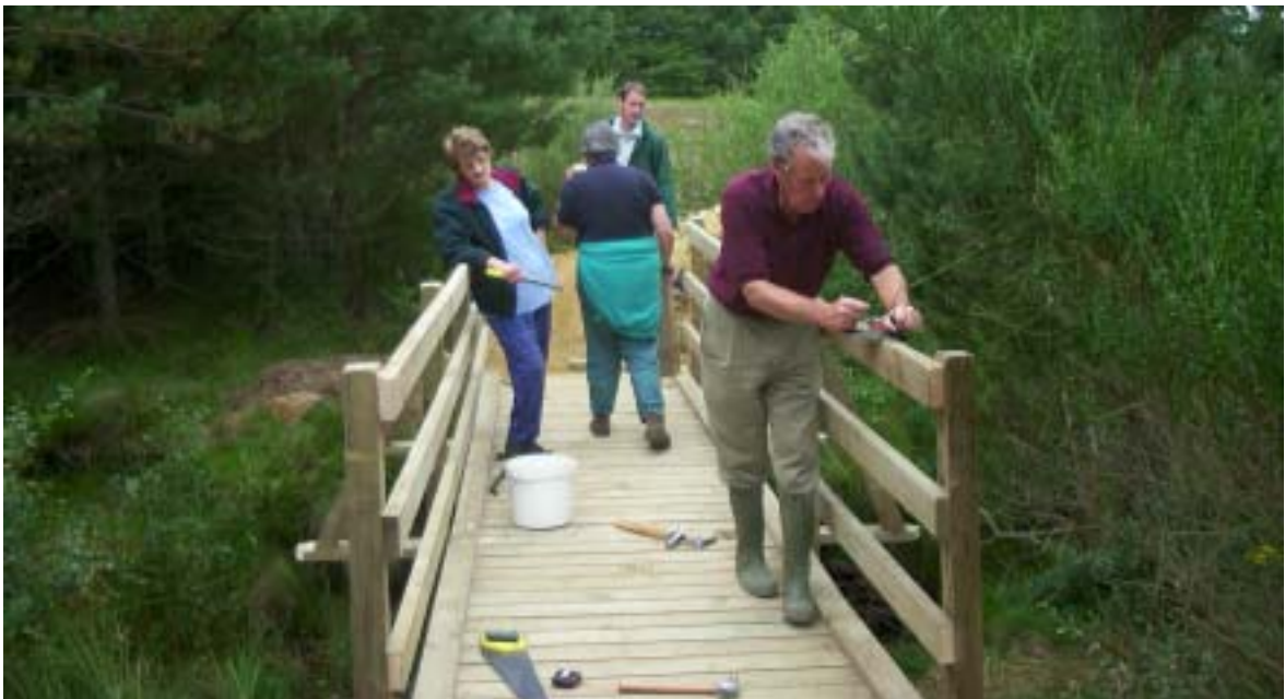
Finishing off one of the bridges
